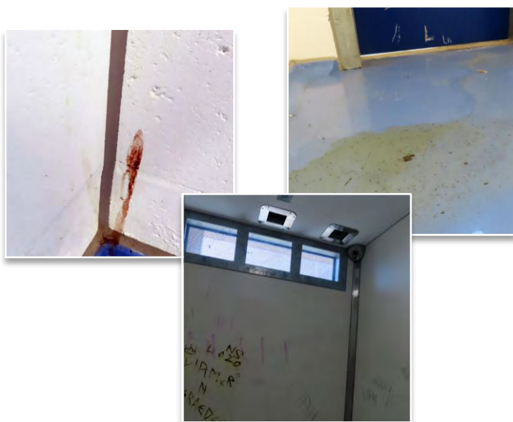
Photos from the on-site inspection of Brisbane YDC.
